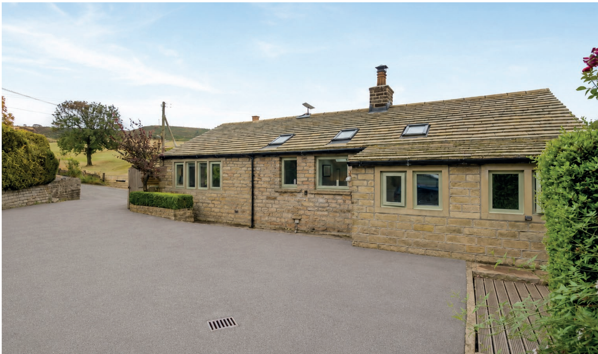
Gatehead Cottage Barnside Lane | Hepworth | Holmfirth | West Yorkshire | HD9 1TN
