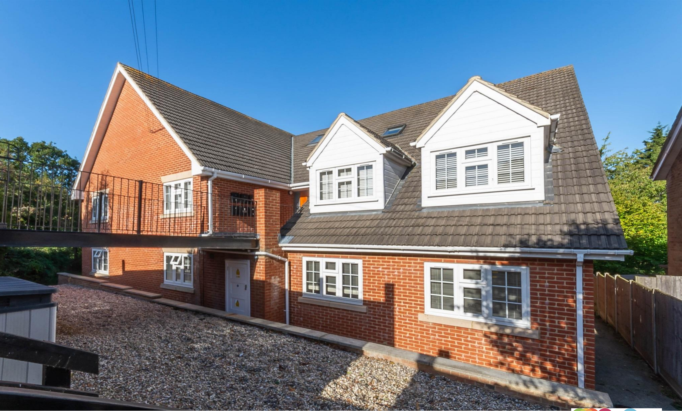
Beacon Hill Court Beacon Hill, Maldon CM9 6HR
