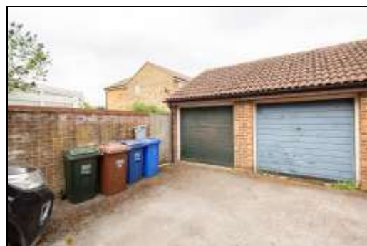
Garage and Driveway Parking
