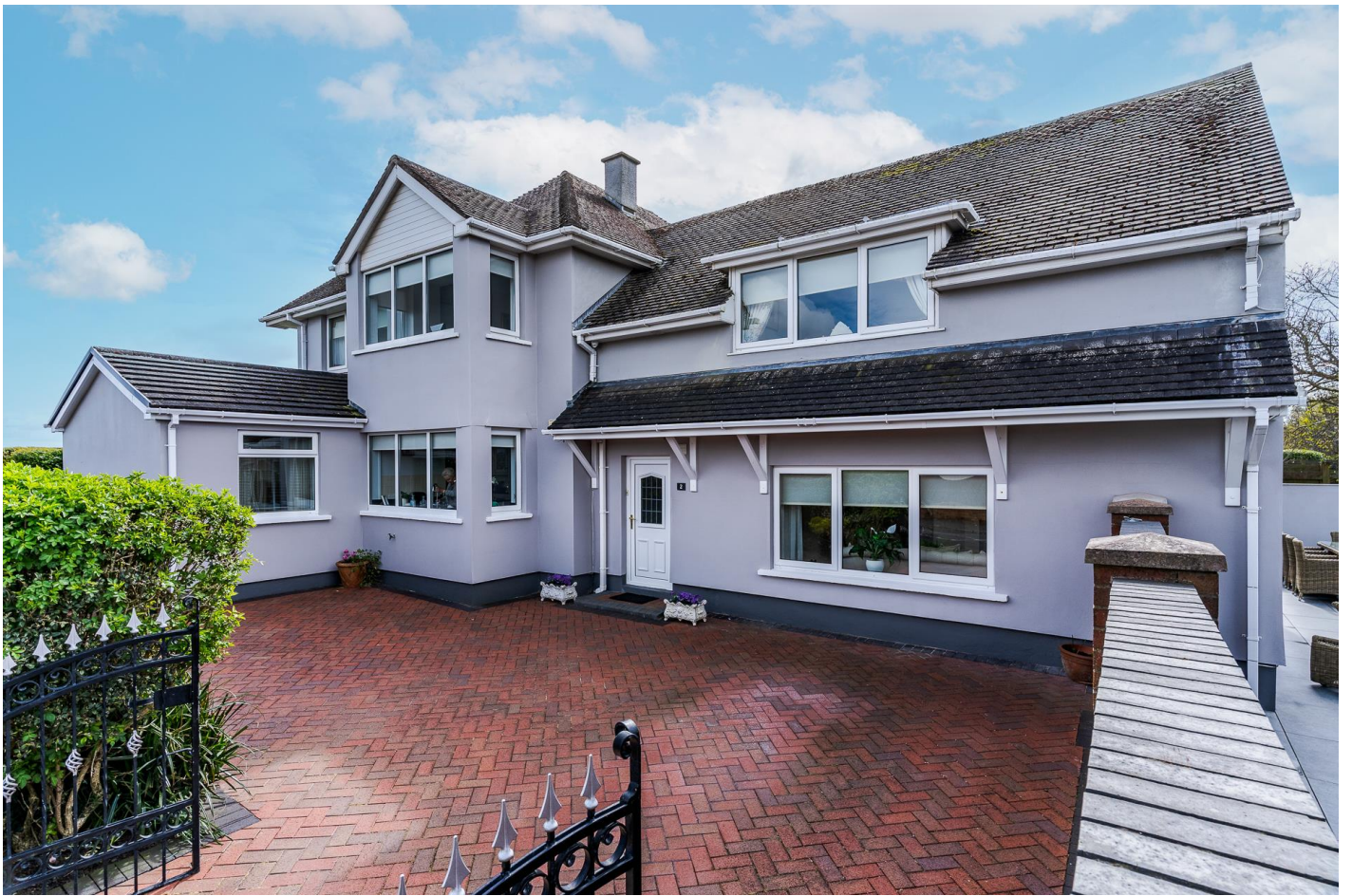
Whitcliffe House, 2 Whitcliffe Drive, Penarth, The Vale Of Glamorgan, CF64 5RY
