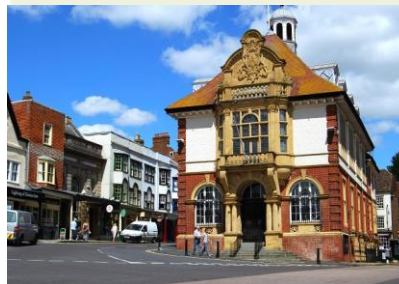
Marlborough Town Hall
