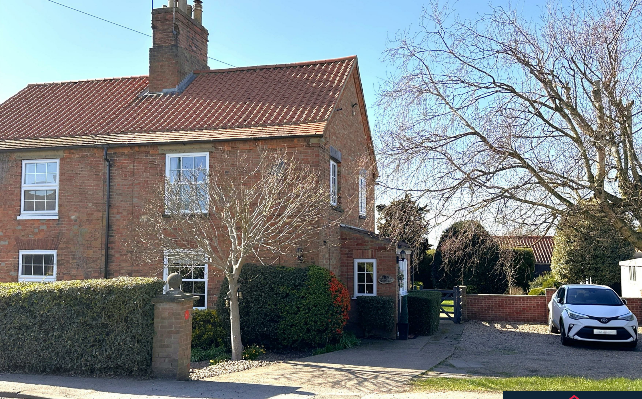
Fleet Cottage, Gainsborough Road, Langford, Newark
