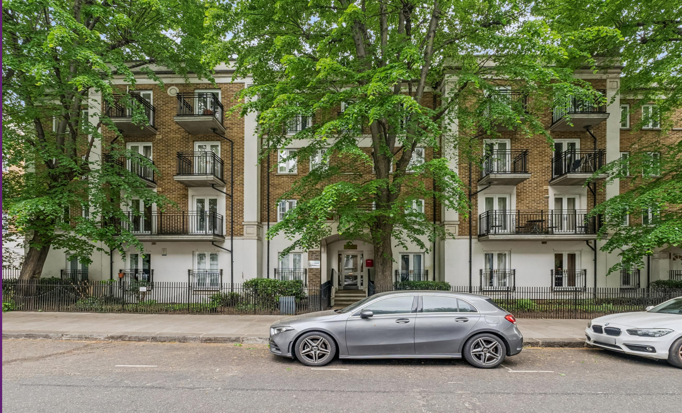
Shillingstone House Kensington, W14
