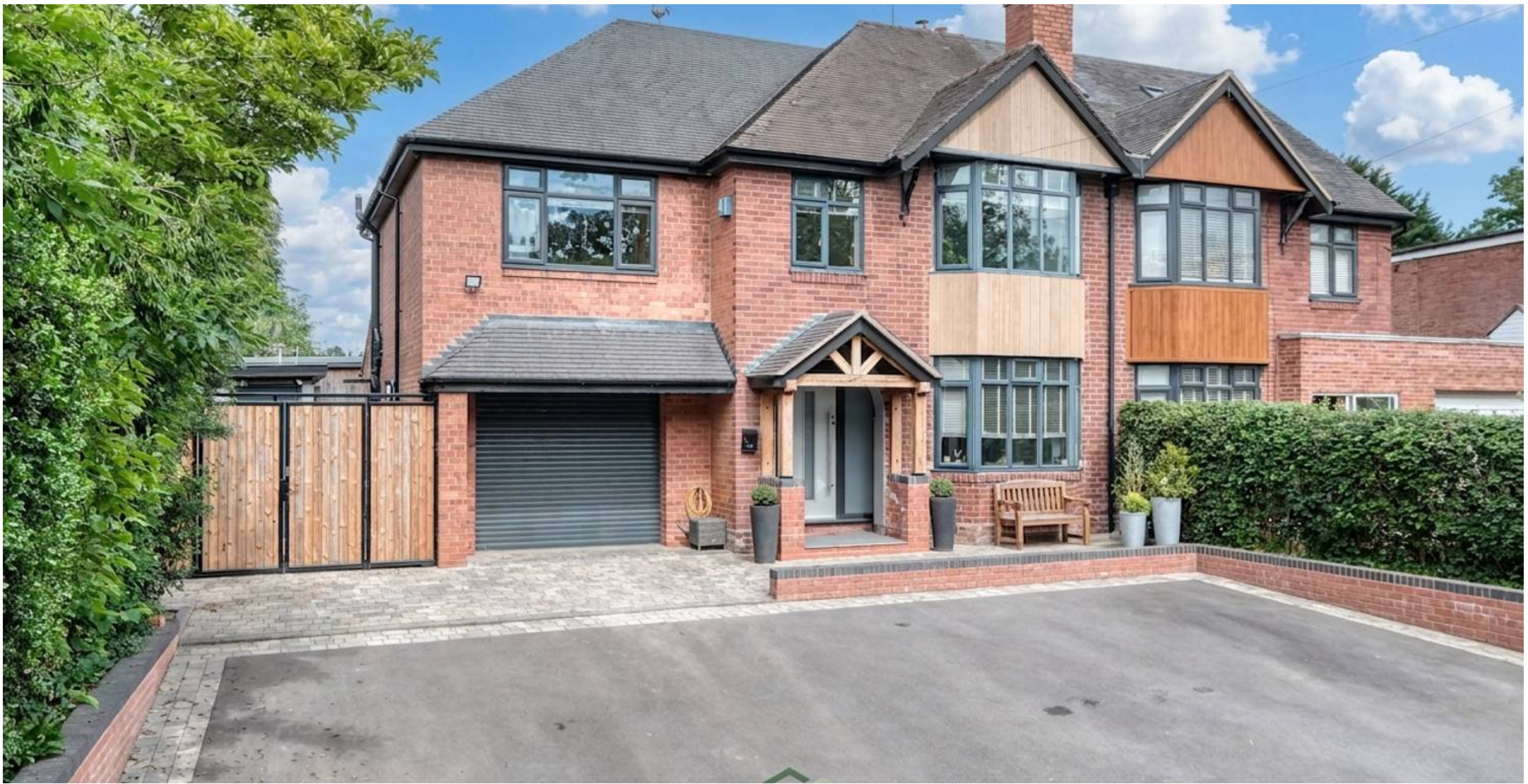
41 St. Godwalds Road, Bromsgrove Bromsgrove
