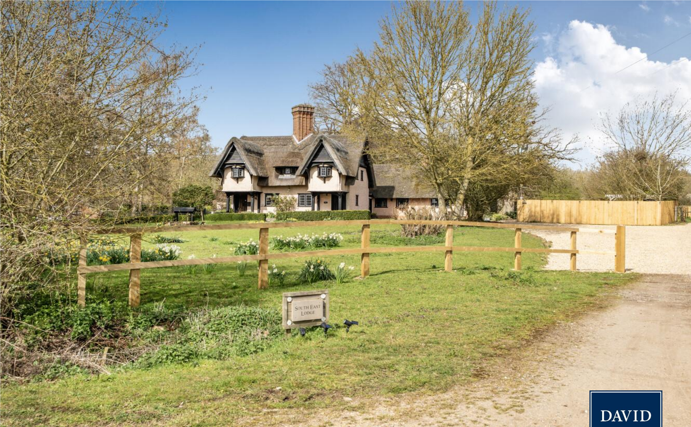
South East Lodge, Whepstead, Suffolk.
