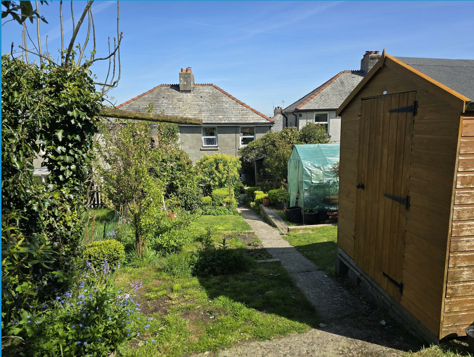
14 Bounsalls Lane Launceston | Cornwall
