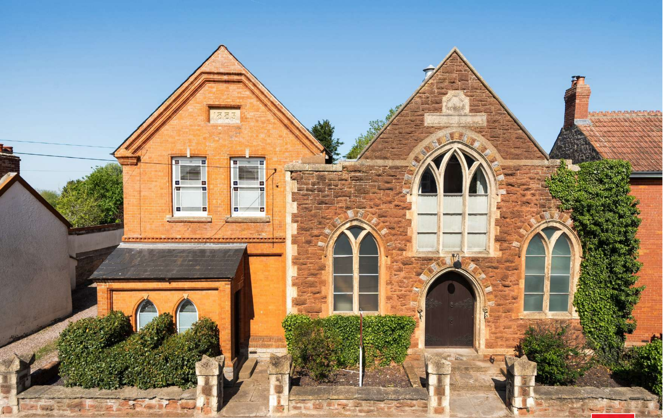
The Old Chapel Fore Street, Othery TA7 0QH
