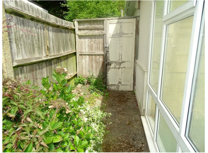
SIDE ACCESS VIEW
