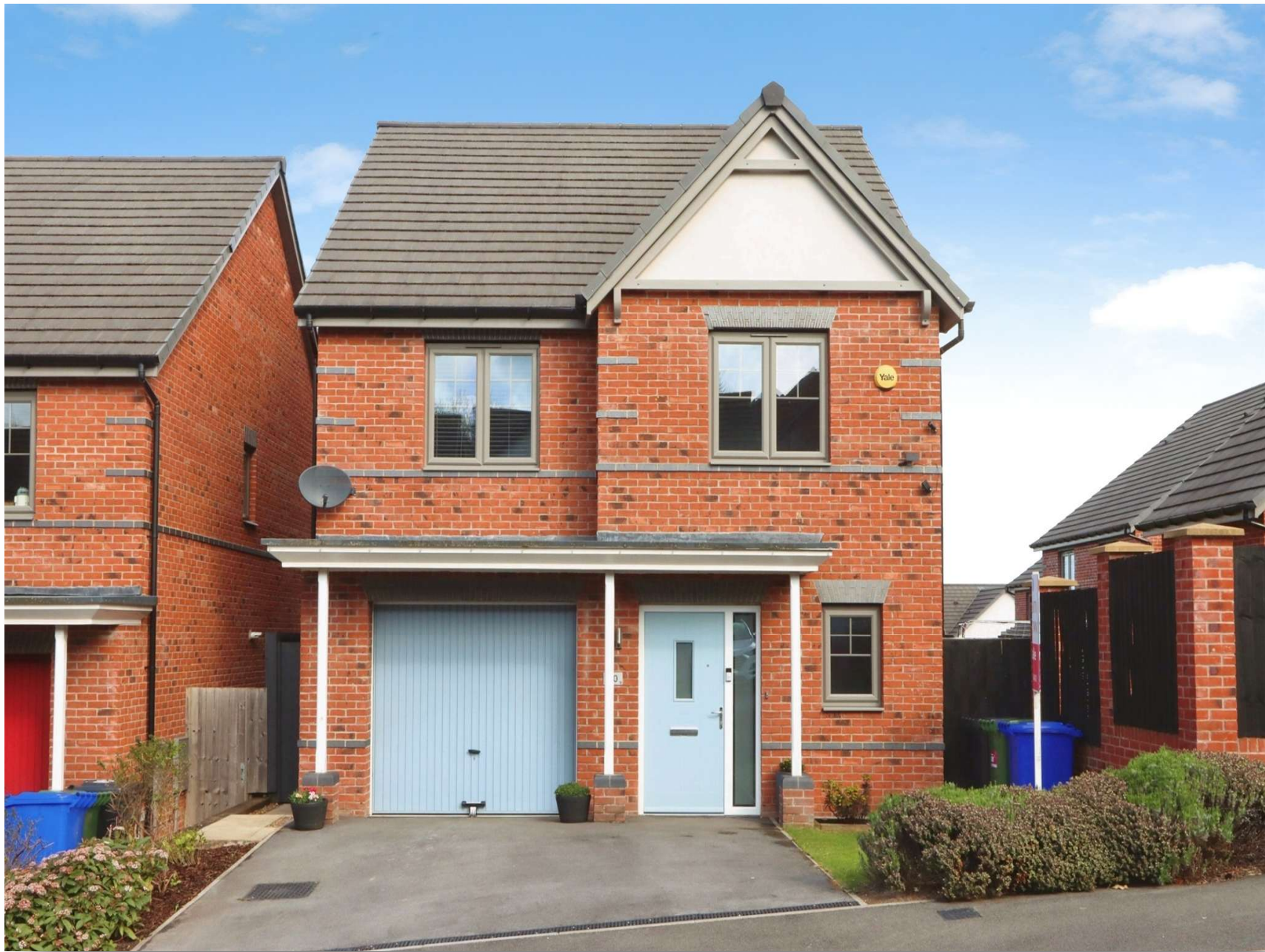
Cranleigh Road, Mastin Moor Chesterfield S43 3BH
