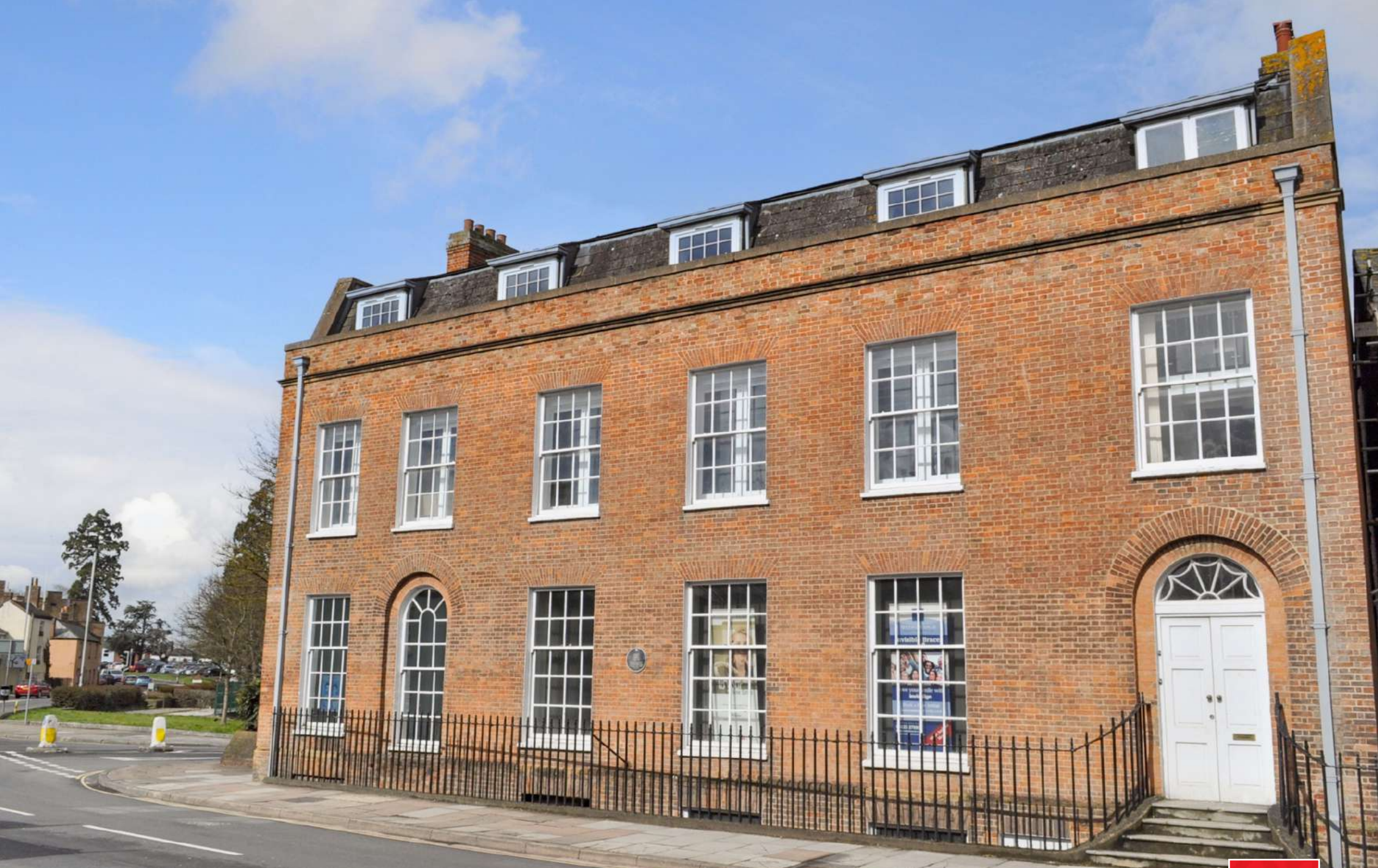
1 General Gordon House The Crescent, Taunton TA1 4BP
