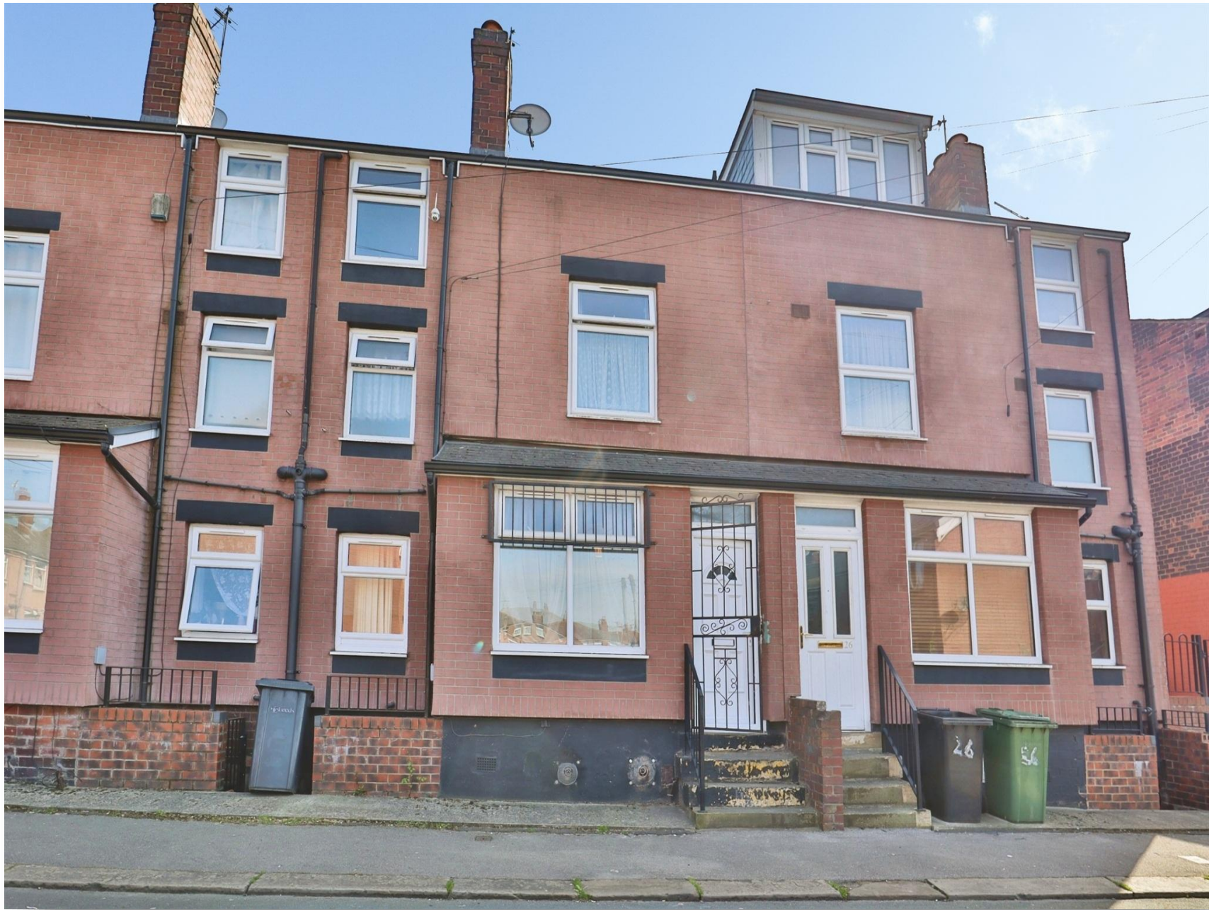
Copperfield View, Leeds LS9 0BJ
