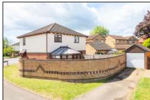
Garage and Driveway
