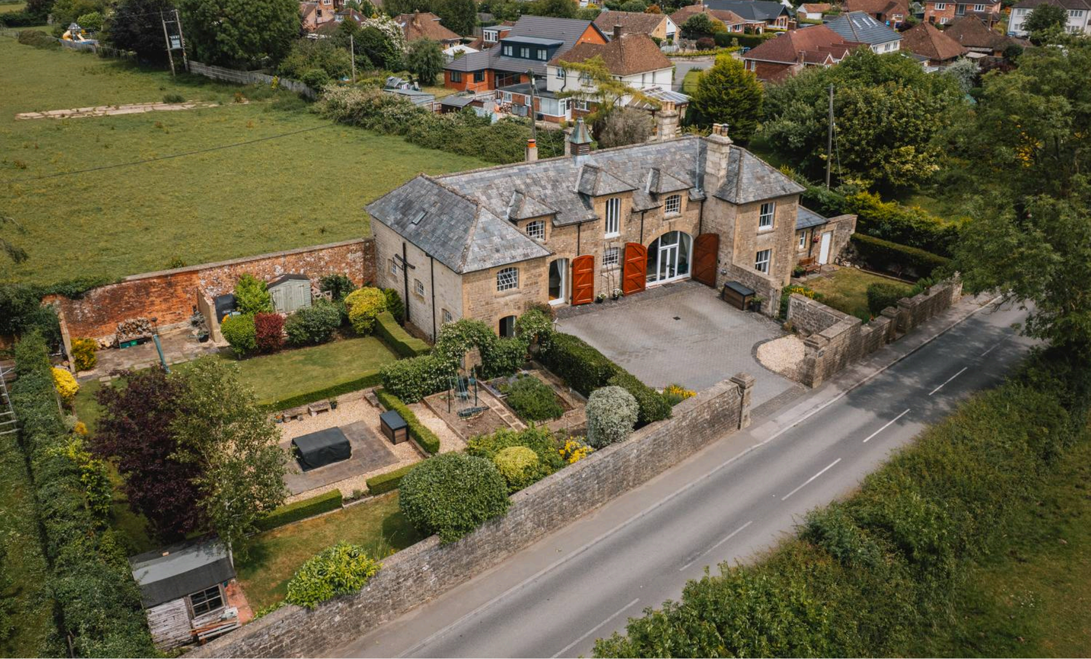
Stable Cottage, 19 Lydiard Green, Lydiard Millicent Wiltshire
