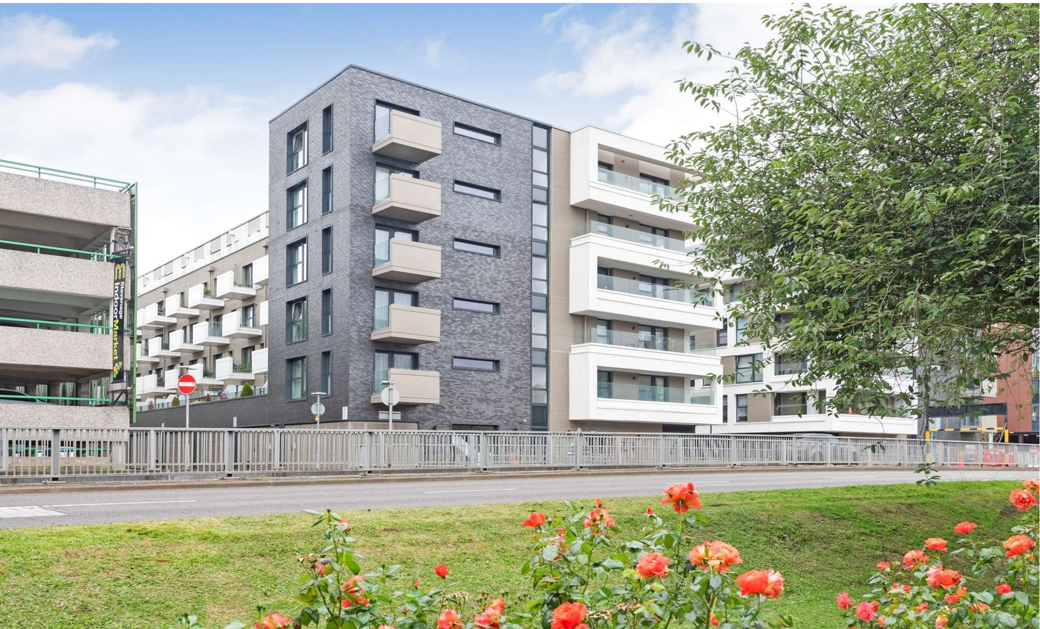
Mulberry House Park Place, Stevenage, SG1 1BH
