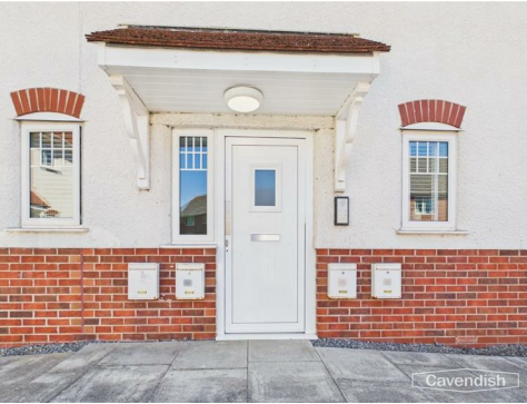
Communal entrance door with intercom entry system.
