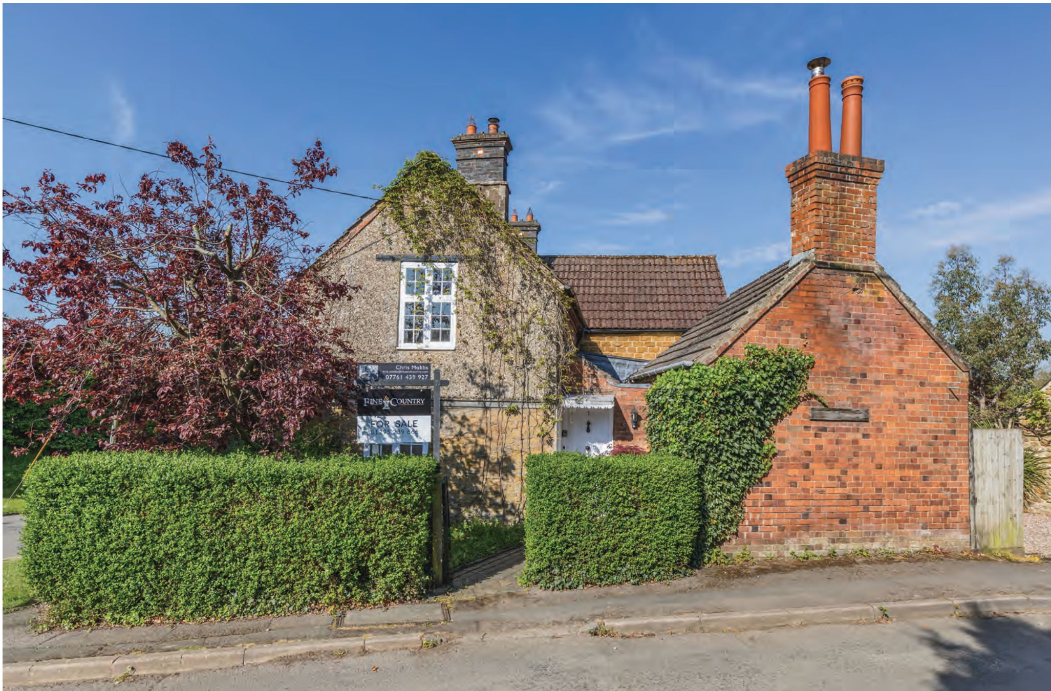
A handsome detached Grade II listed period house in this popular village. The extended cottage offers four reception rooms (three with open fireplaces), kitchen, cellar, three to four bedrooms, family bathroom, shower room, some new double-glazing, LPG central heating. There is a 26m by 7.5m private garden, on road parking and no chain. Full of character is a great village.
