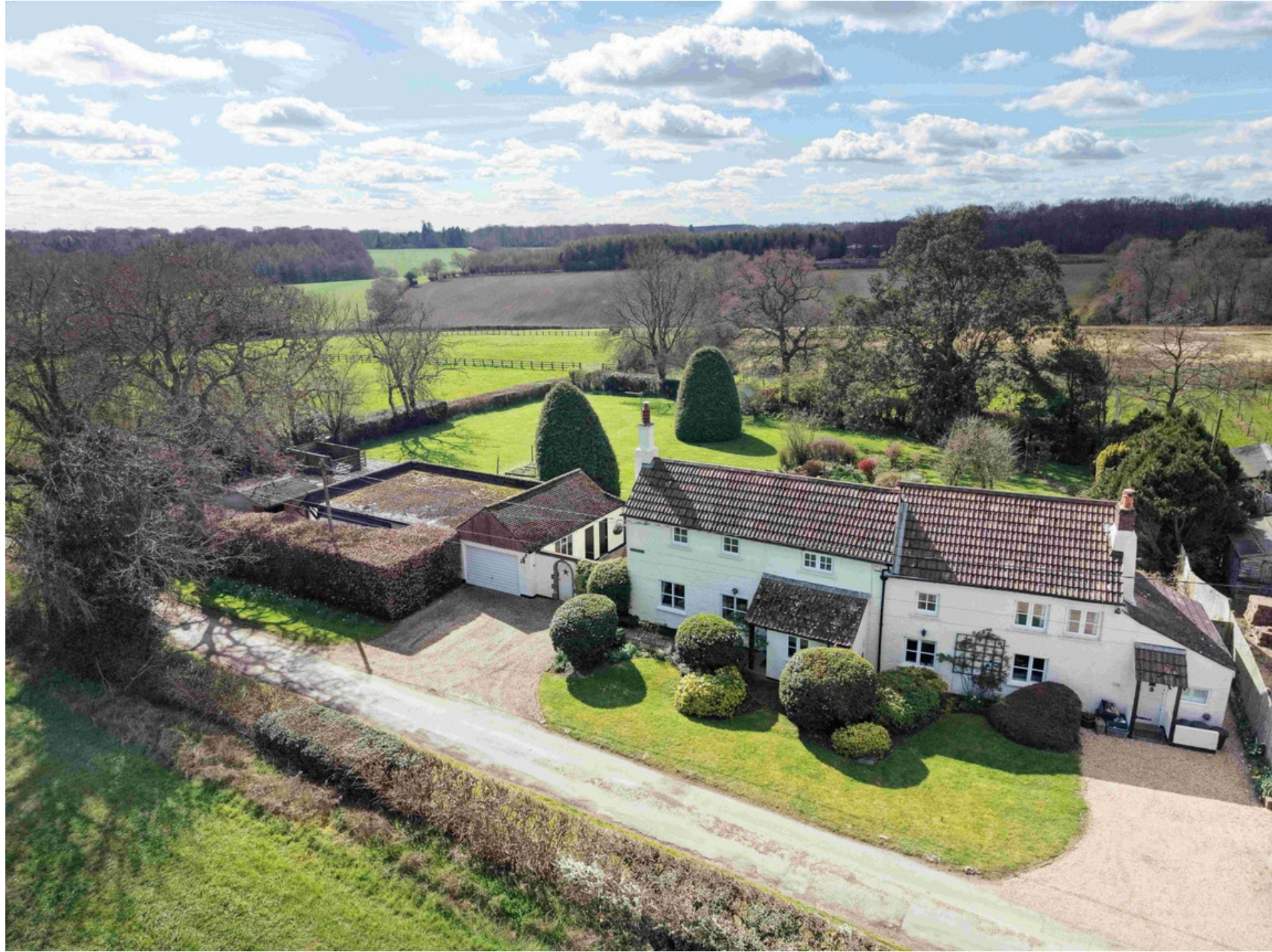
CORFIELD, ARREWIG LANE, CHESHAM
