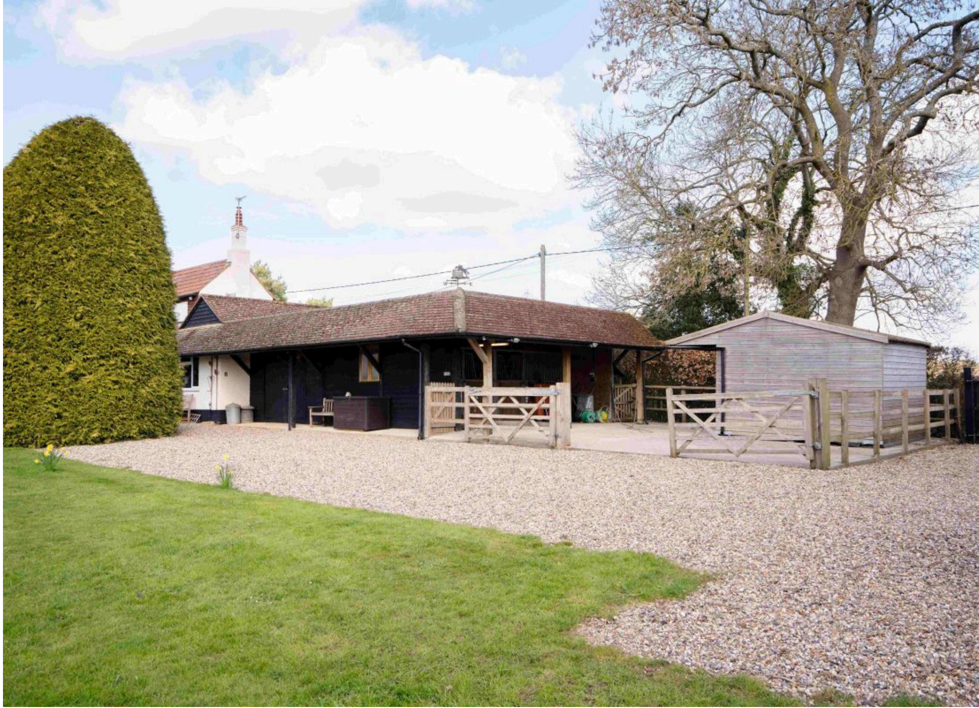
CORFIELD, ARREWIG LANE, CHESHAM
