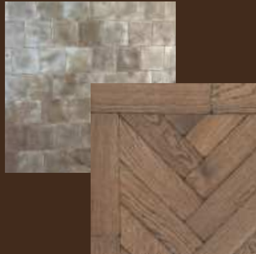
Original glazed wall tiles and restored parquet flooring
