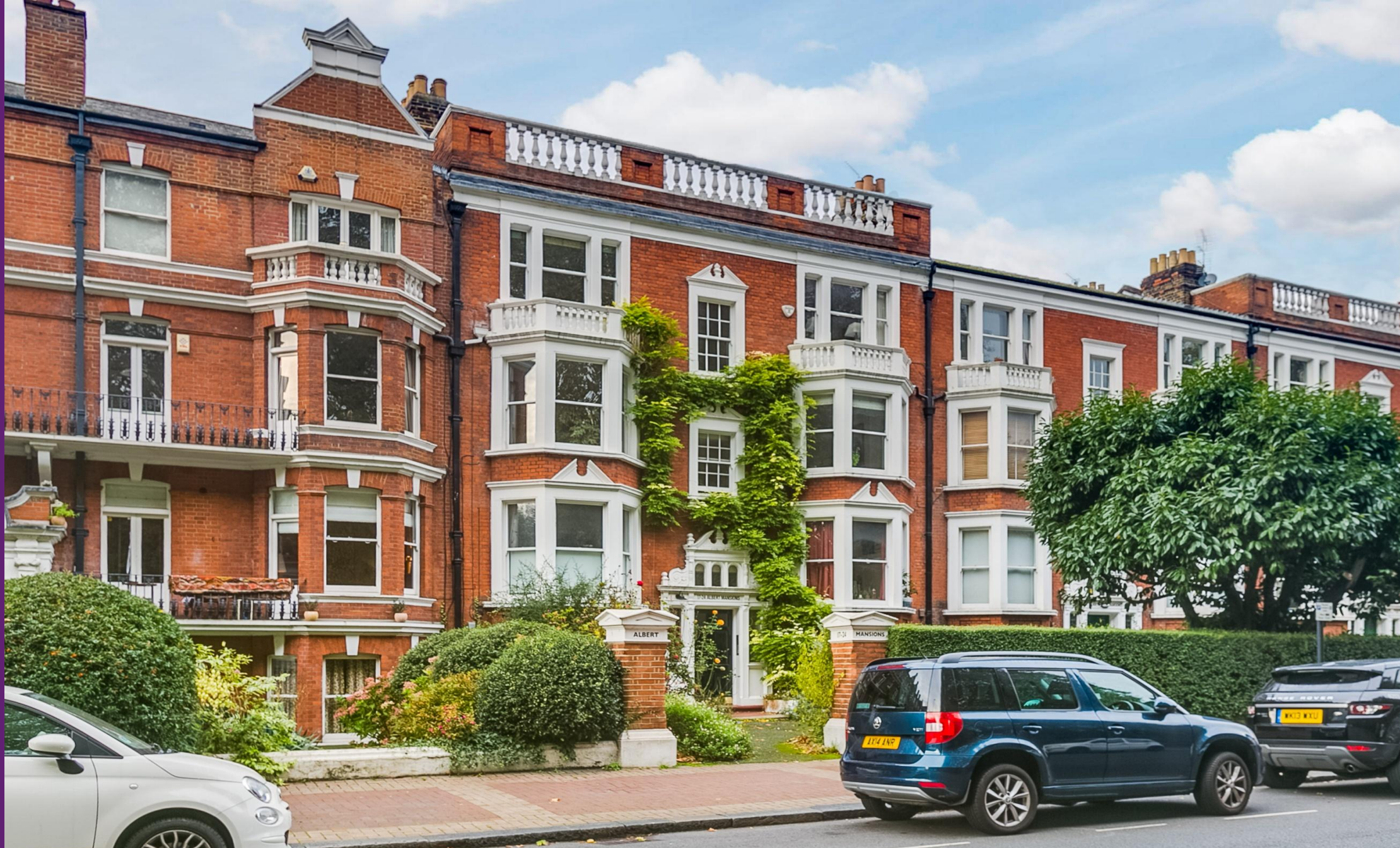
Albert Mansions Albert Bridge Road, SW11
