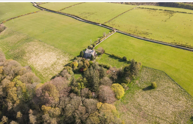
Aerial photo of Spring House
