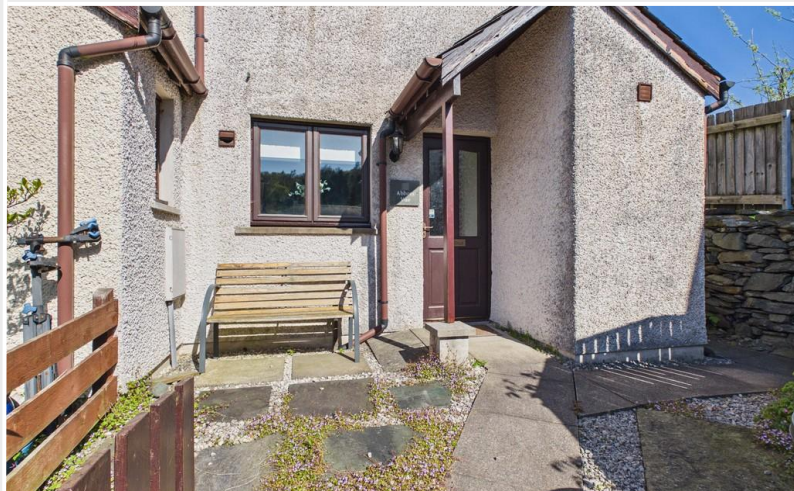
Front Entrance and Forcourt Garden
