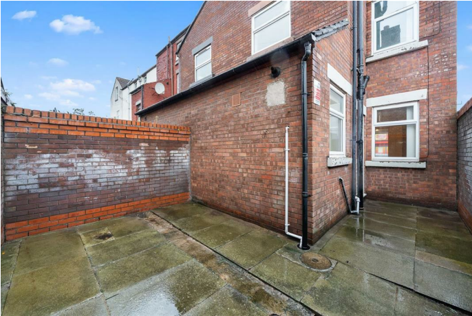
walled yard with gated access to side aspect
