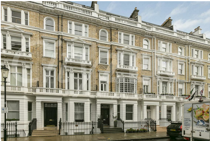
EXTERNAL OF BUILDING
