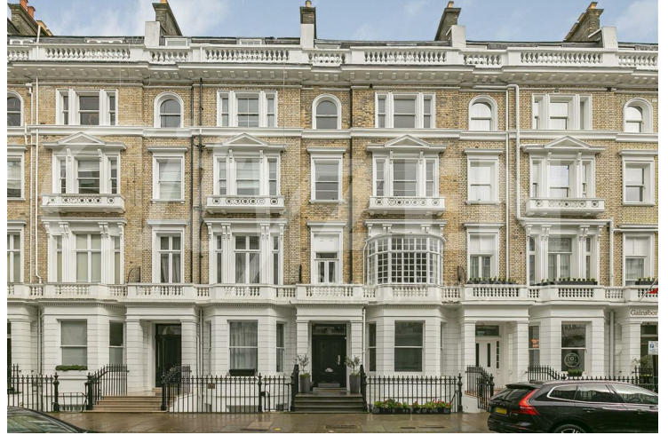
EXTERNAL OF BUILDING
