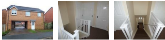
UPVC entrance door, double glazed UPVC window, two radiators, power and light points
