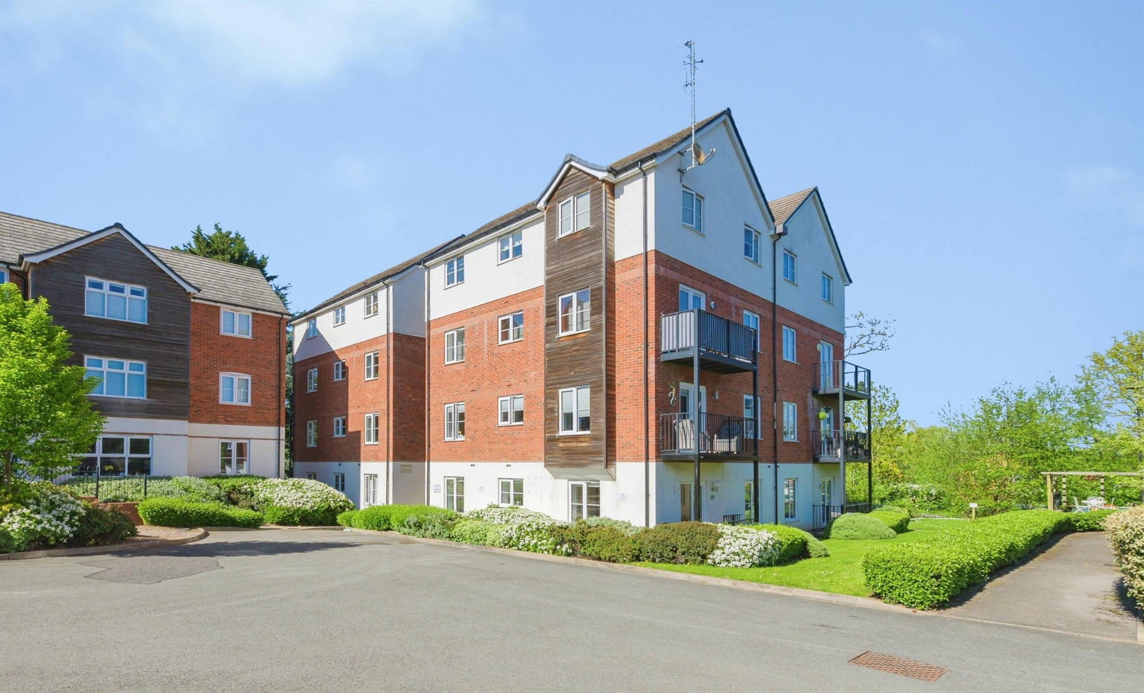
Fielding House, The Laurels, Fazeley, TAMWORTH
