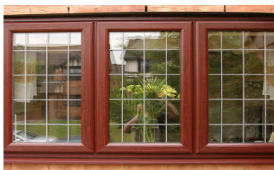
3 Timber framed brown painted windows
