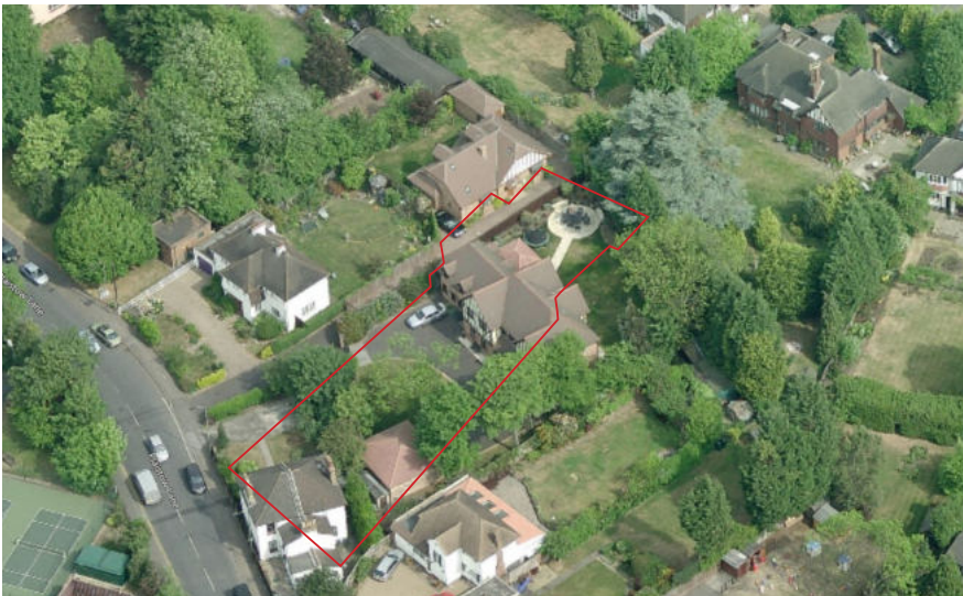
Birds-Eye View of the site looking from the South-West
