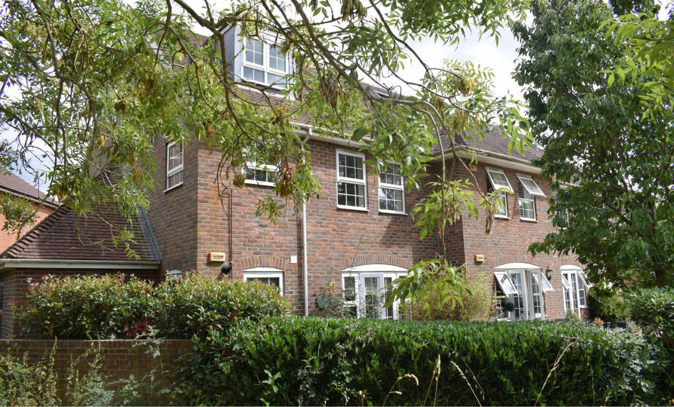
Yeoman Court, Reigate Road, Burgh Heath Tadworth
