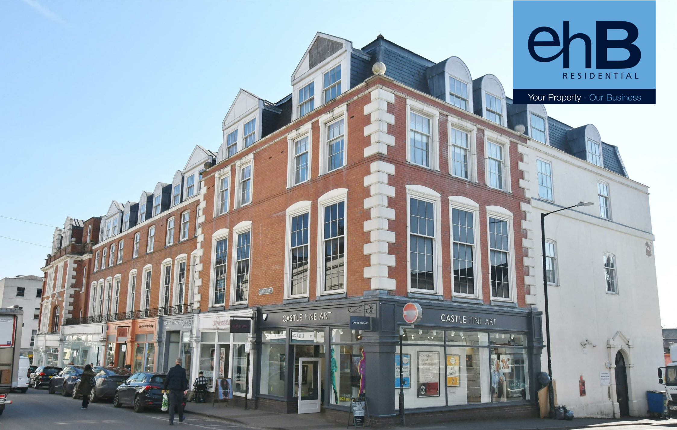
Apt 18 Woodward House, 43 Bedford Street, Leamington Spa
