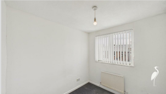
Double glazed window rear and radiator.
