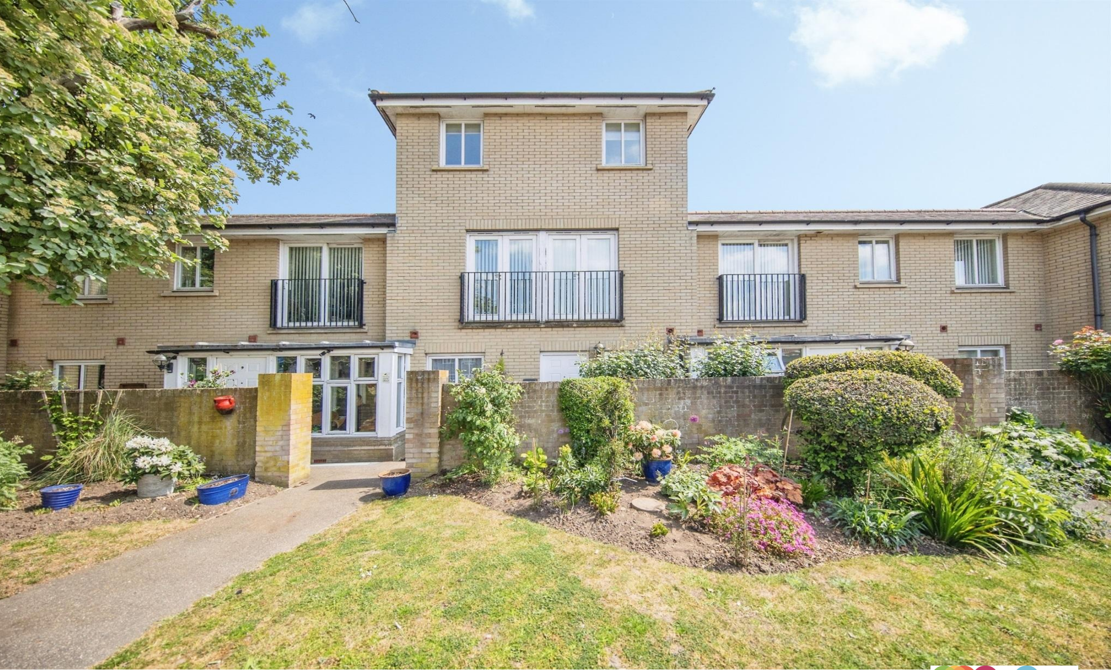
Croft Court, Gregory Street, Sudbury CO10 1HE
