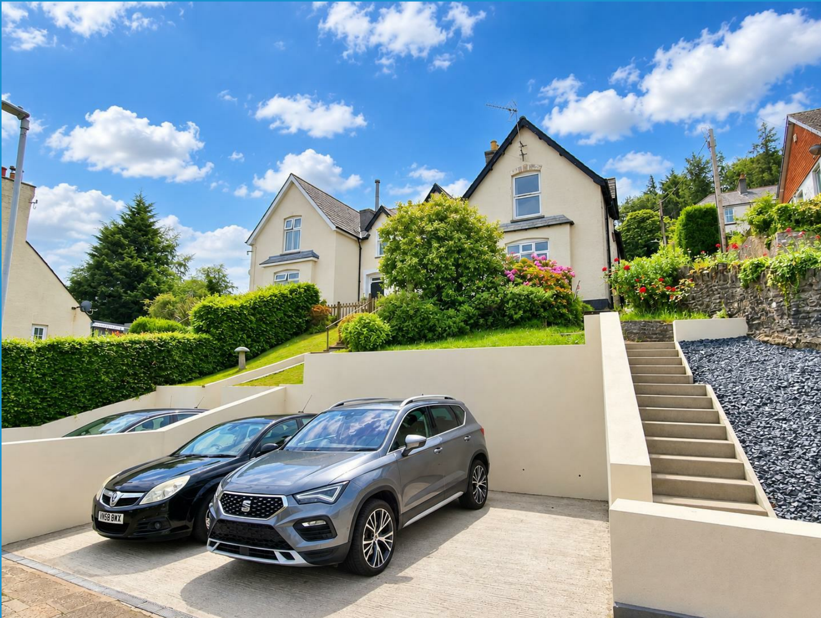
3 Westgate Terrace Launceston | Cornwall
