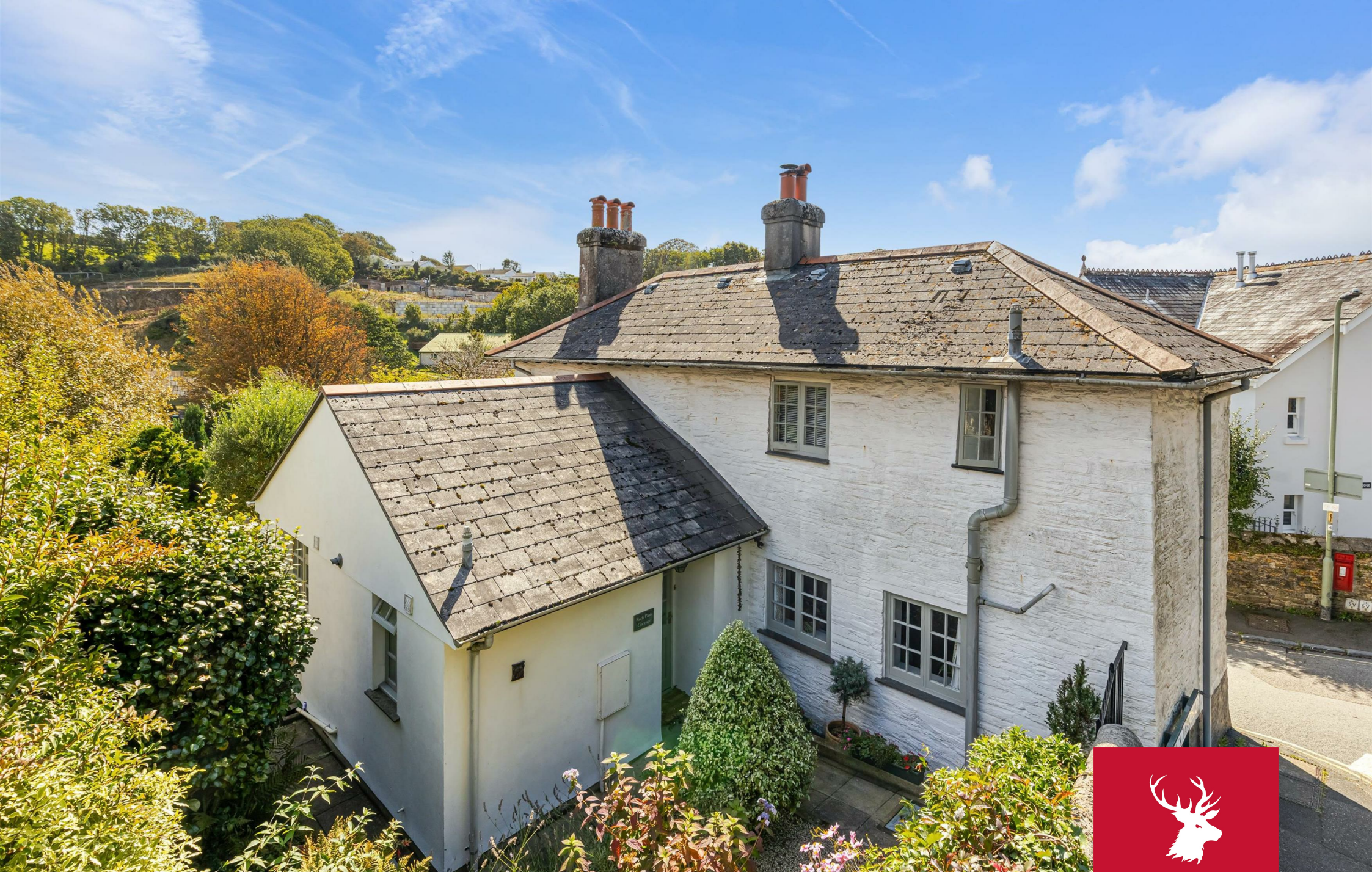
Rack Park Cottage
