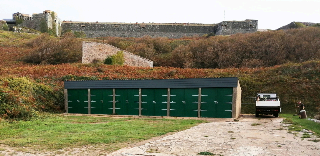
Garage 4 block built garage with double opening doors.
