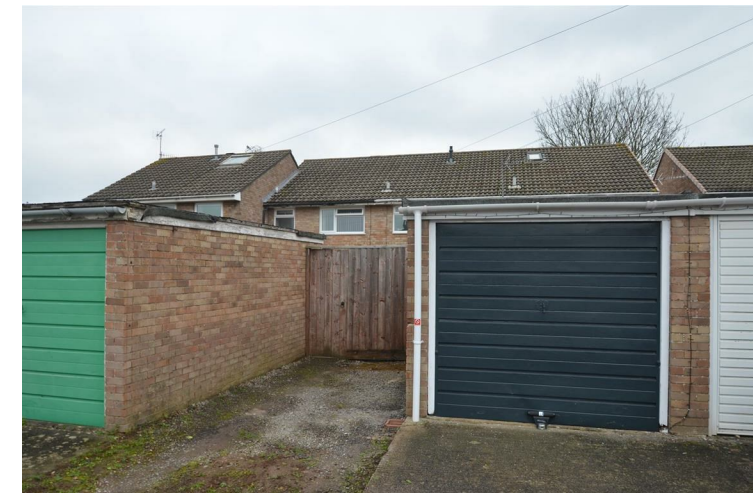
Accessed via an up and over door. Light and power connected.
