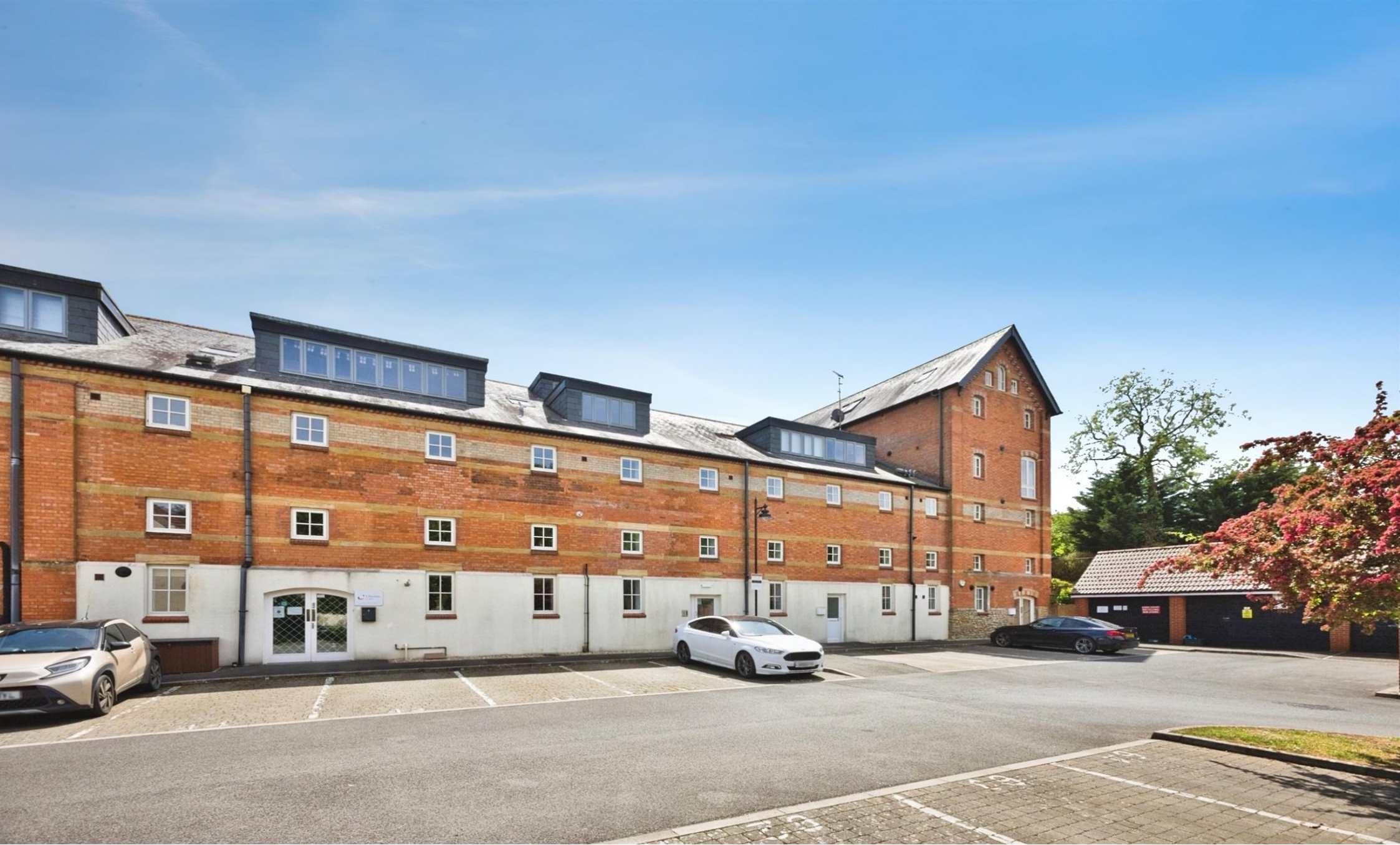
The Barley Yard, Old Mill Lane, Crewkerne TA18 7BQ
