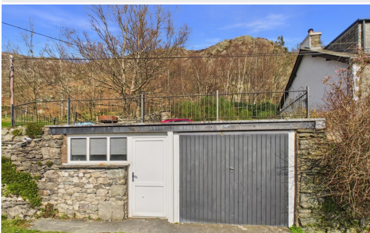
Workshop and Garage
