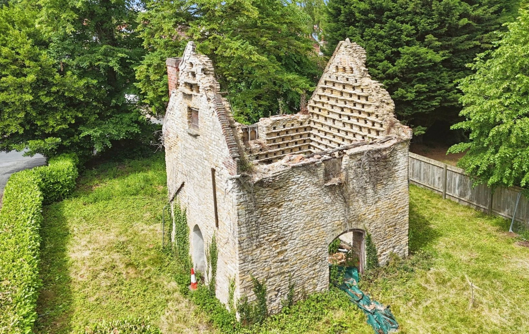
The Dovecote – Development Opportunity, South of 44 Main Street, Elloughton
