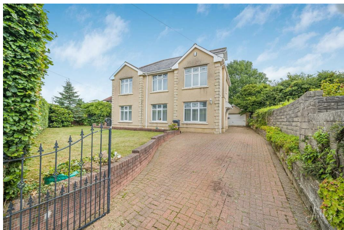
Main dwelling view
