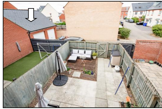
Overview of the Garden & Garage (white arrow) from the Juliette Balcony on the French doors
