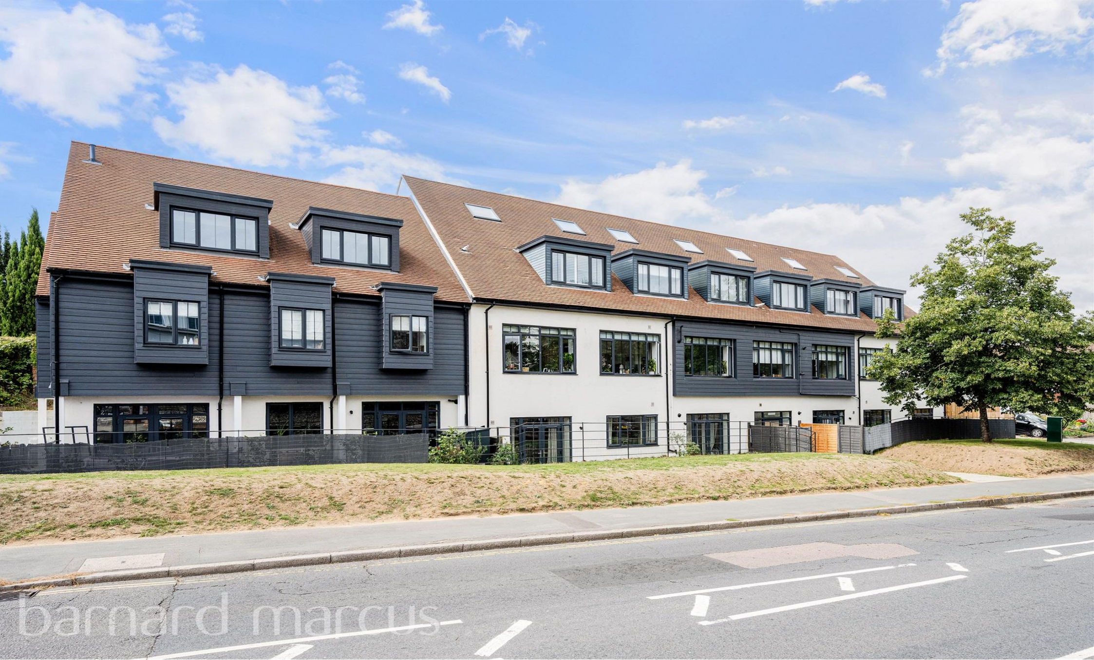
Mulberry House, Station Road, Dorking RH4 1EB
