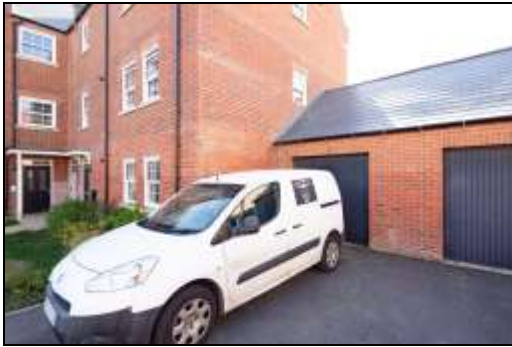
Garage and Driveway Parking
