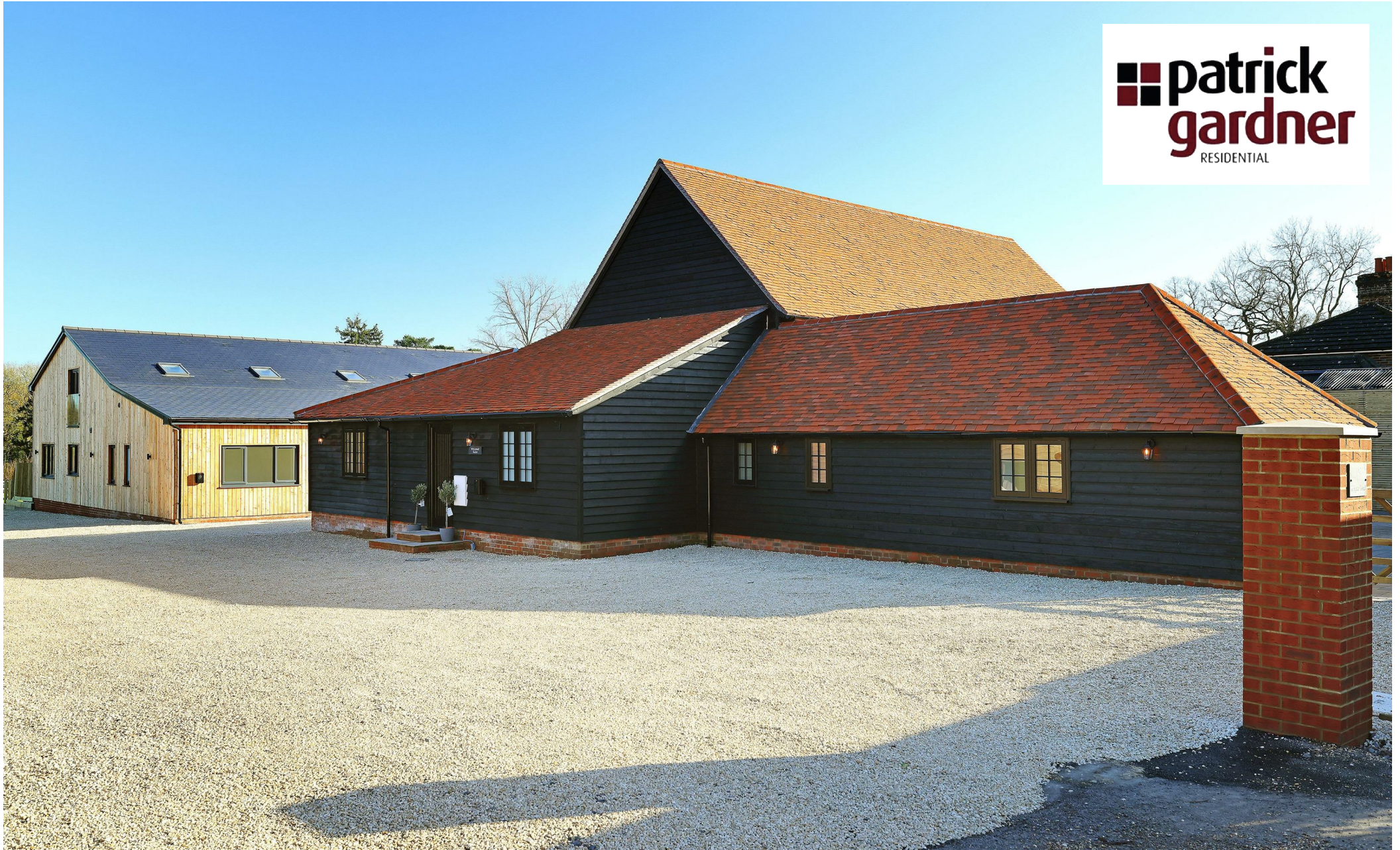
Williams Barn, 15a Reigate Road, Sidlow, Surrey, RH2 8QH
