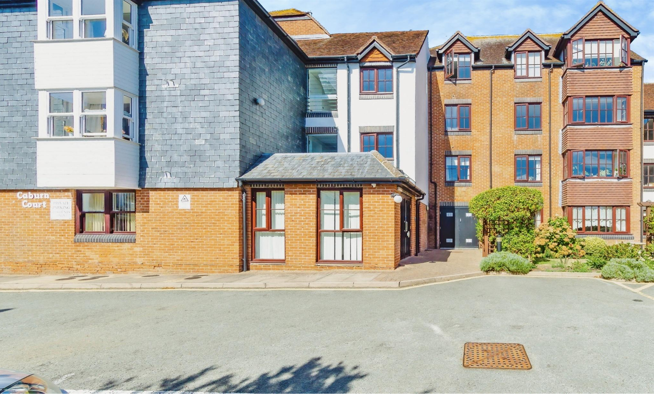
Caburn Court Station Street, Lewes BN7 2DA
