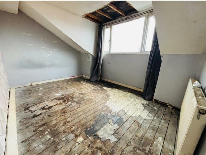
Double glazed window, central heating radiator
