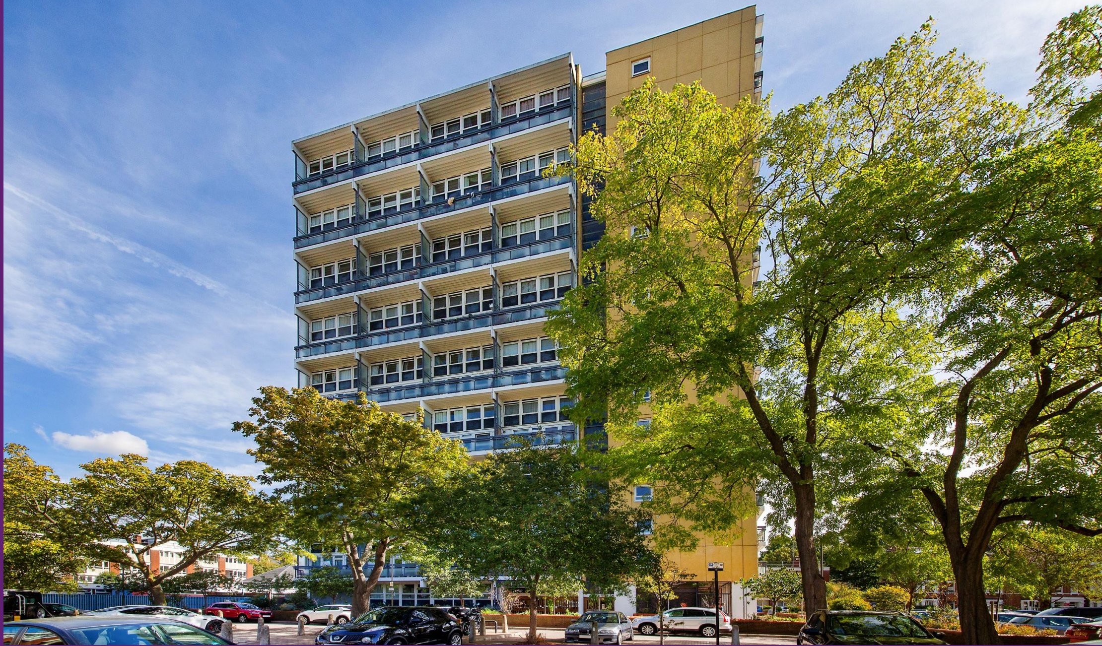
Ethelburga Tower Rosenau Road, SW11
