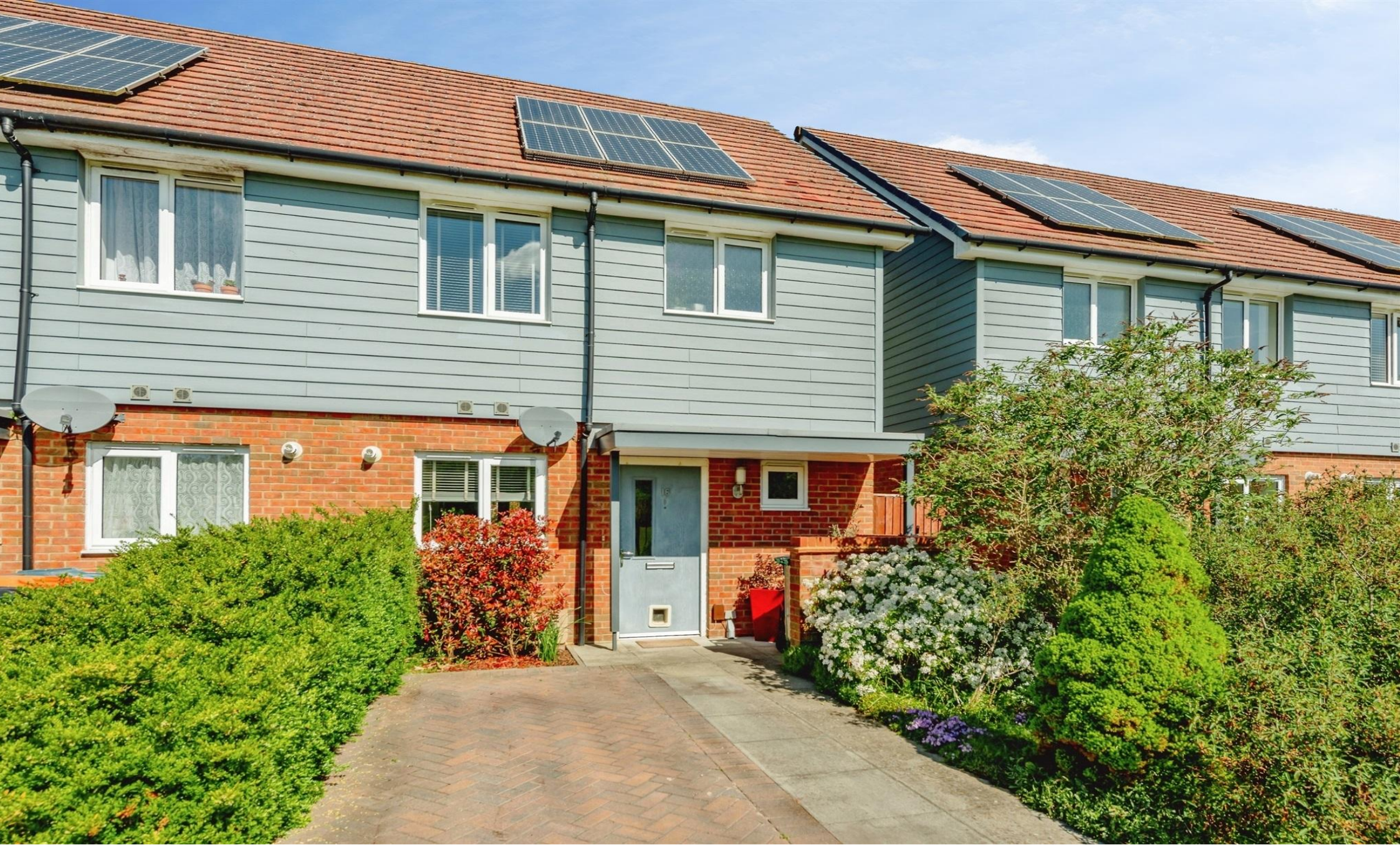
Waterfall Crescent, Bewbush Crawley RH11 8WA
